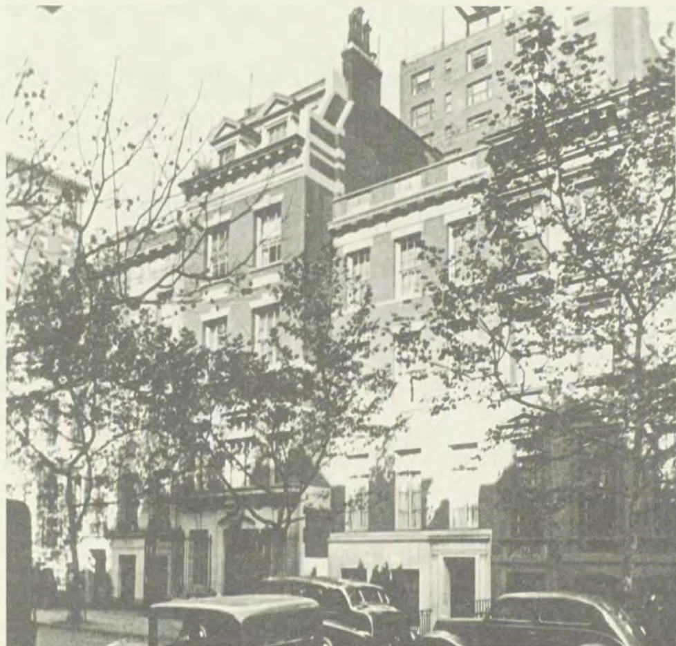
Figure 16. Arthur Bourne House (center), 117 East 55th Street, 1939.
